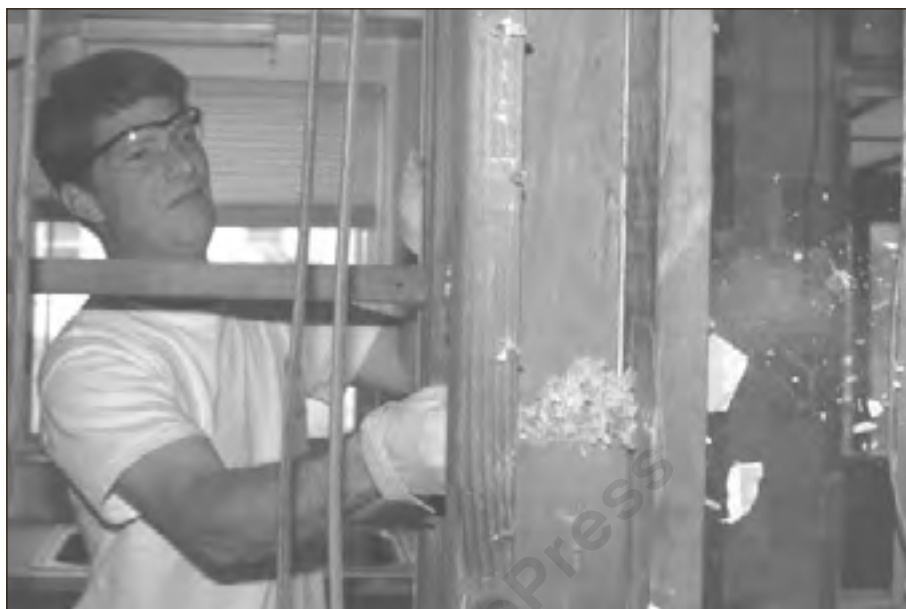
Ken Midkiff of North uses a hammer to knock down Sheetrock that had been damaged by the hurricanes.
